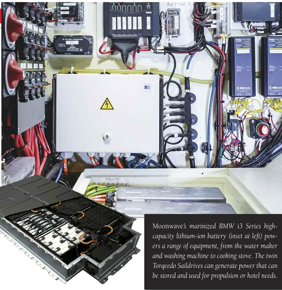
Moonwave's maritized BMW i3 Series high-capacity lithium-ion battery (inset at left) powers a range of equipment, from the water maker and washing machine to cooking stove. The twin Torqeedo Saildrives can generate power that can be stored and used for propulsion or hotel needs.
